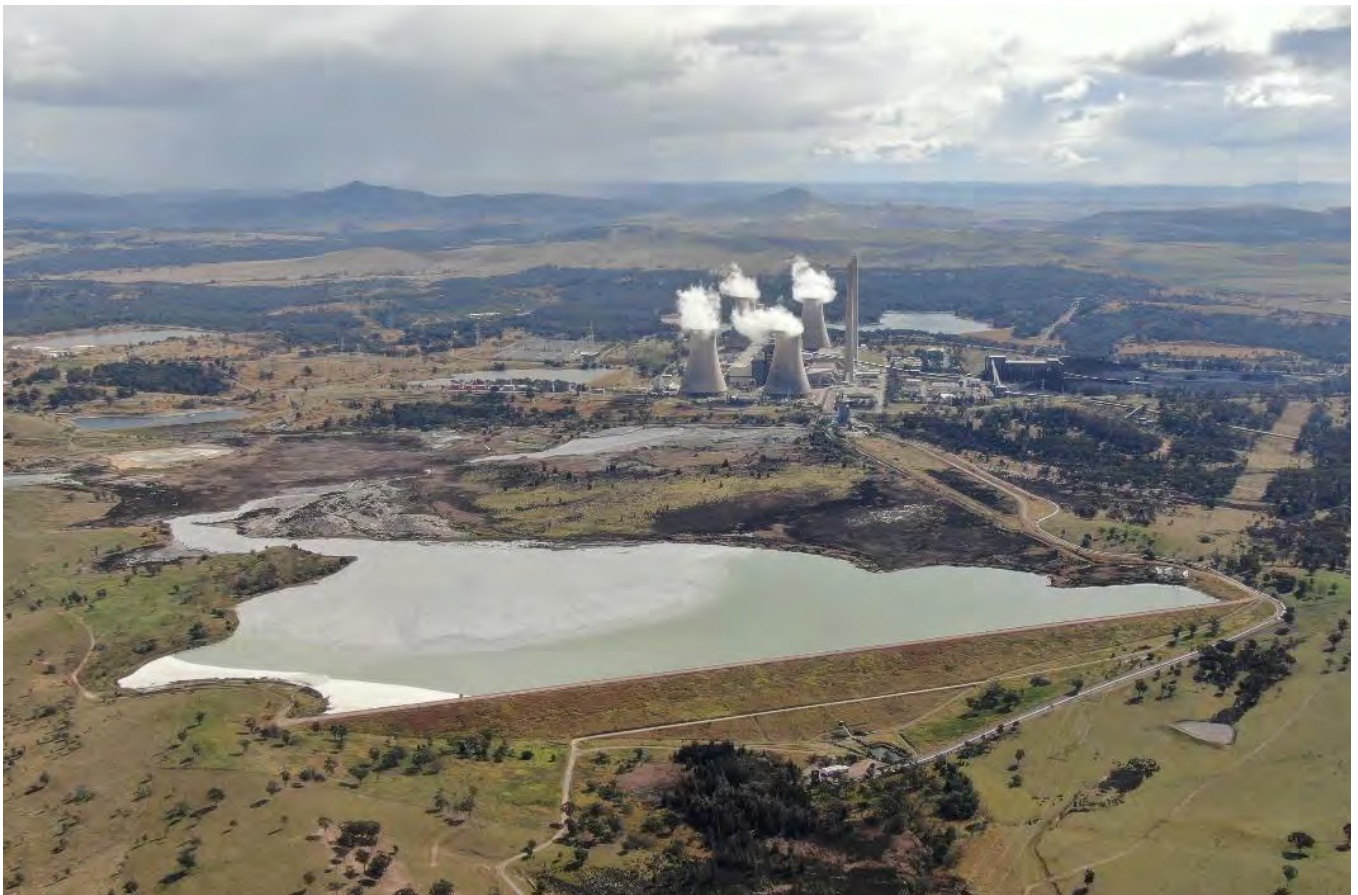
Bayswater power station. HCEC.
