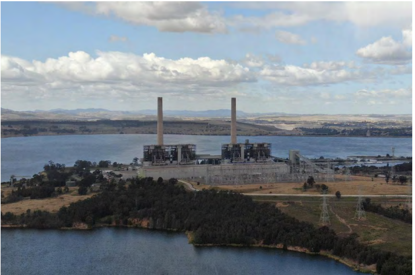
Lake Liddell and Liddell power station. HCEC.
