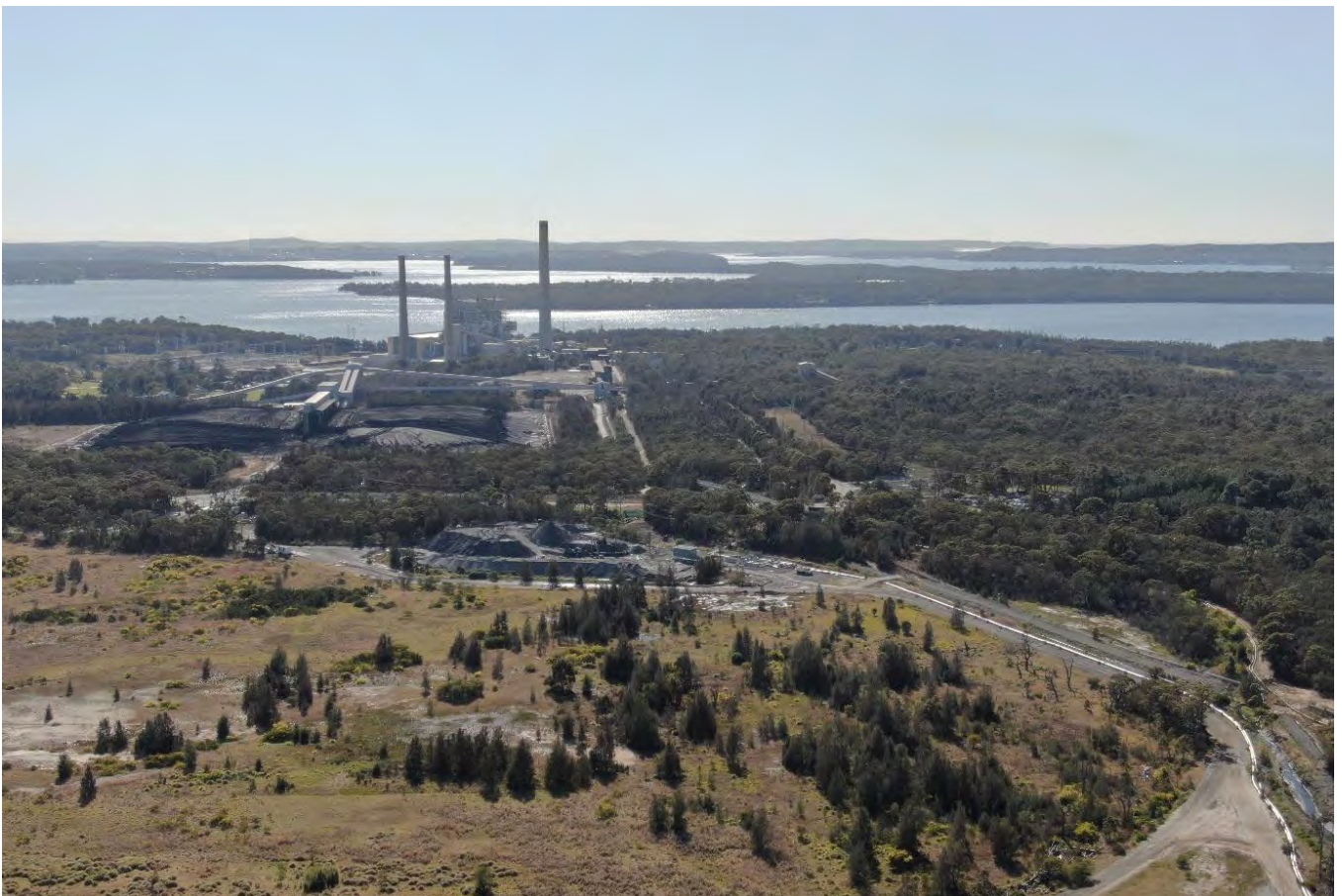
Vales Point power station. HCEC.
