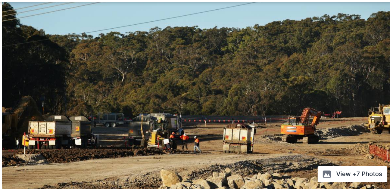
📷 Newcastle Inner City Bypass construction - Pictures by Simone DePeak
