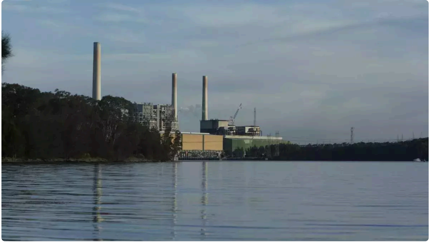
📷 Vales Point Power Station.
